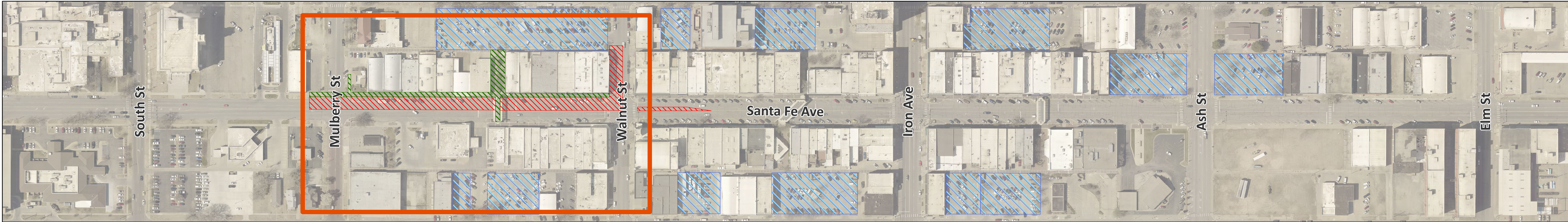
Full Length of Santa Fe Ave. Construction
